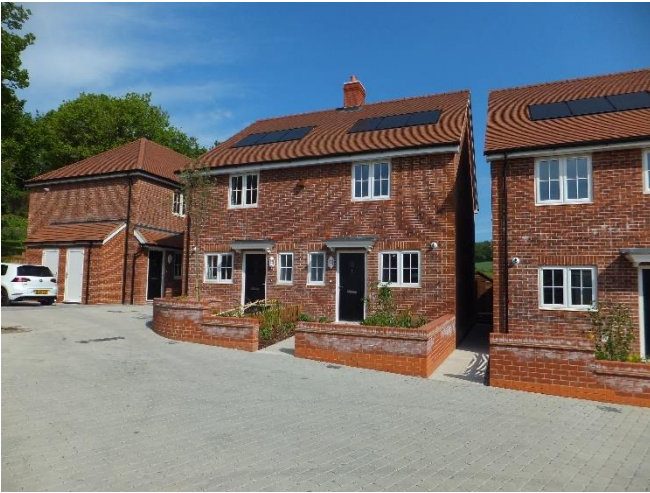
New affordable homes in Midhurst
